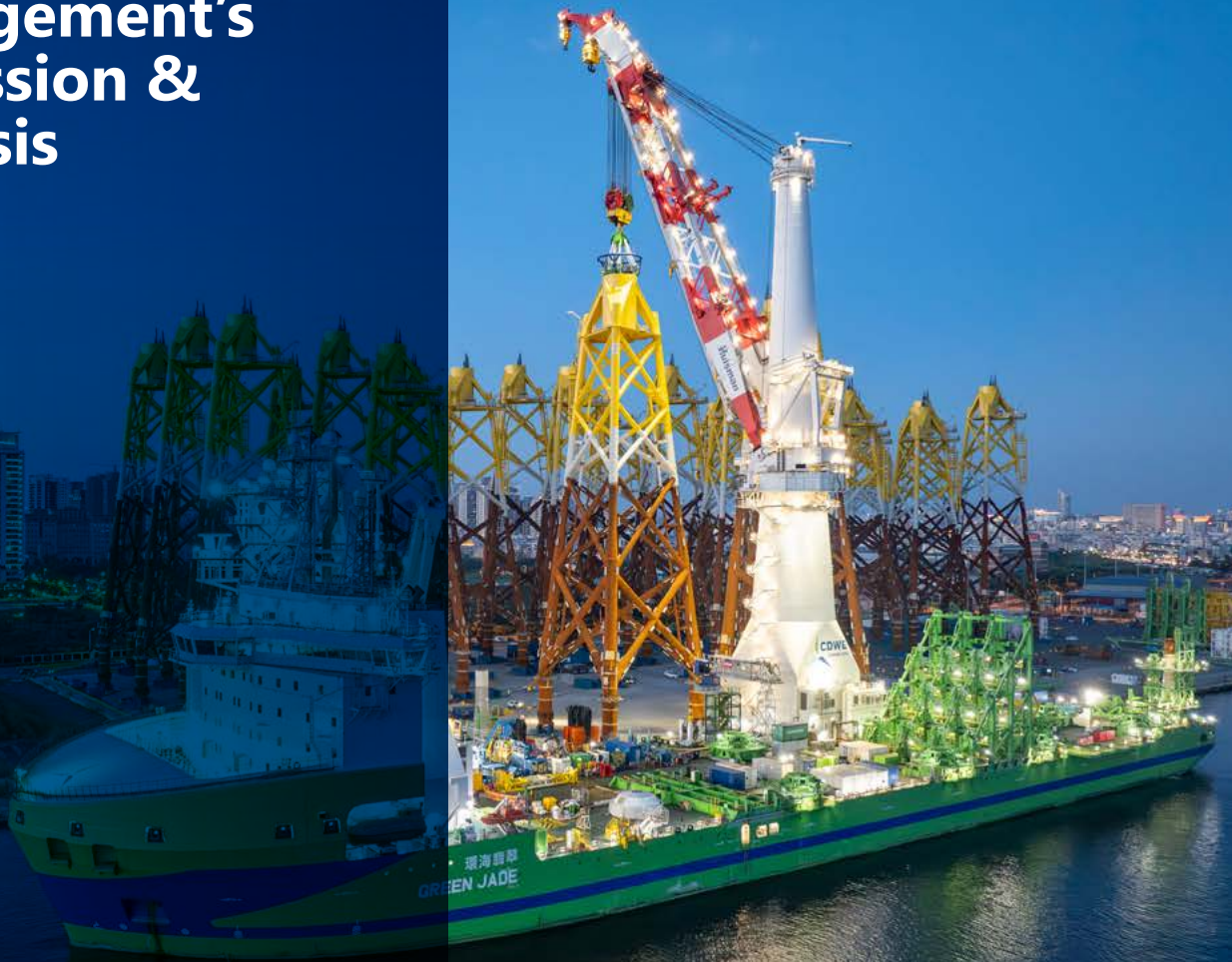
The Green Jade (vessel) loading jacket foundations
