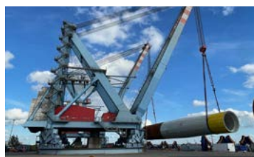
Monopile loadout on the Svanen vessel in Poland.
