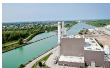
Thorold natural gas facility in Ontario
